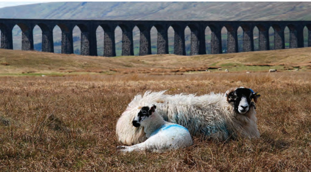
Photo: Ribbleshead Viaduct, by Tanya St. Pierre
